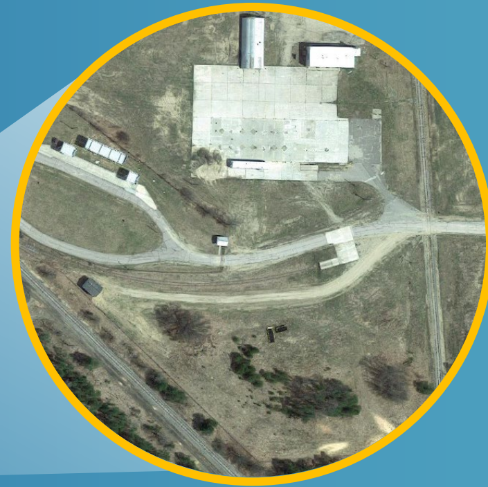
Former Bulk Storage Tanks Location
