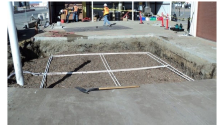
Infiltration Pipe Installation
