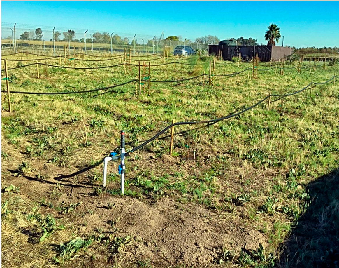
Wetland Irrigation Station and Drip Emitters
