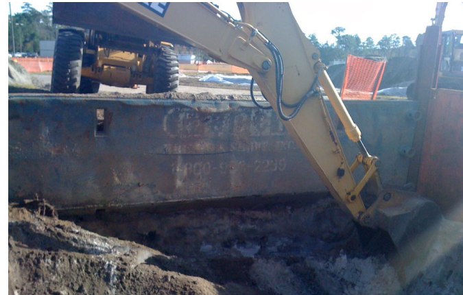
Excavation with shoring
