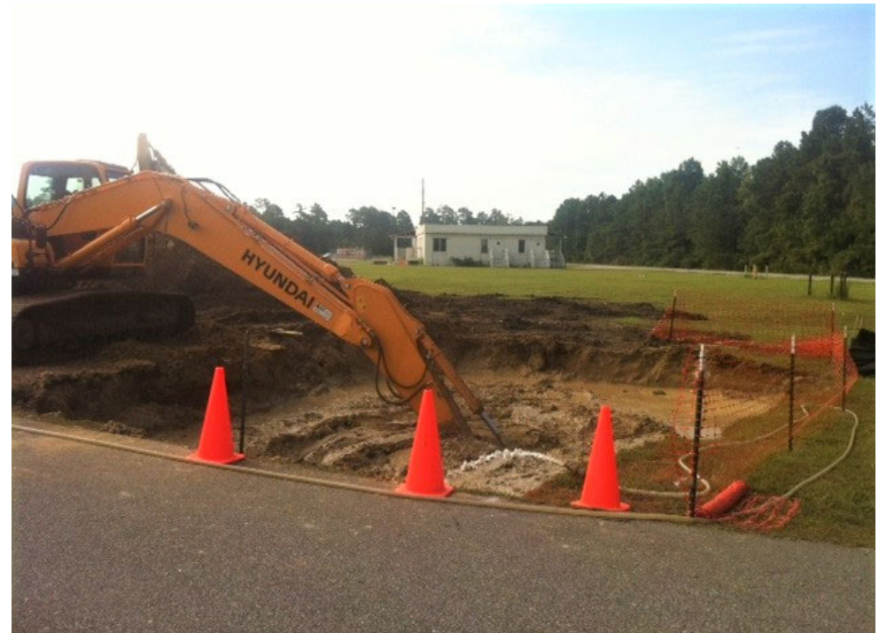
Soil mixing with Persulfate at FOLTA
