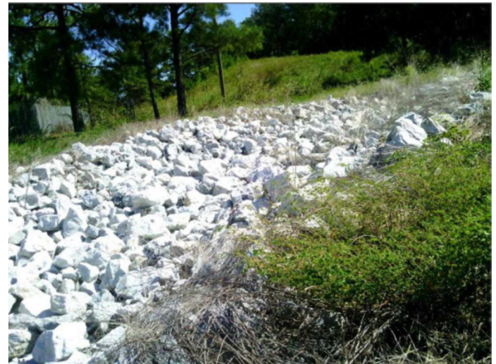
Riprap in ditch near waste pit
