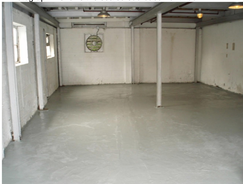
Photograph 1. Sealed Sub-basement Floor
