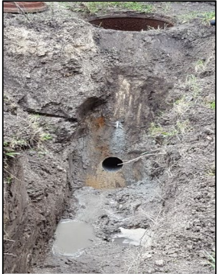
Blower Connection to Manhole
