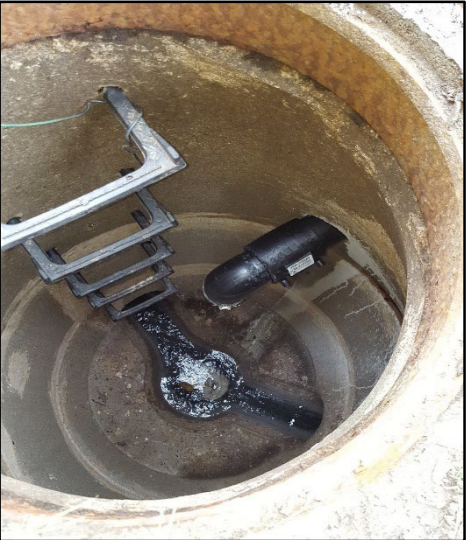
Piping into manhole
