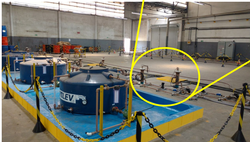
Detail of above ground recirculation wells infrastructure
