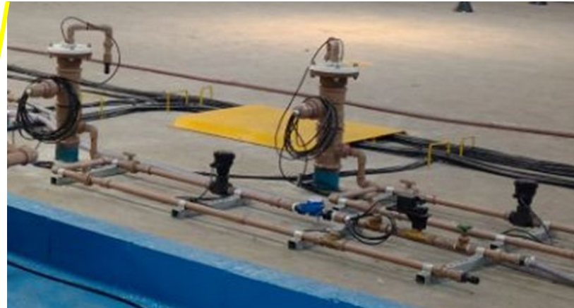
Detail of above ground recirculation wells infrastructure
