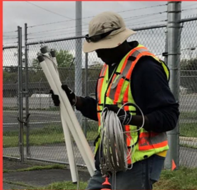
place soil into screened housings
