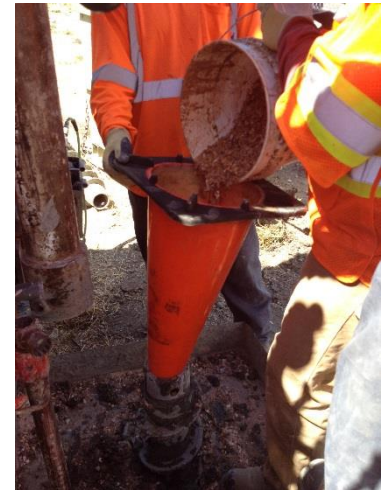
Borings above PFB fill were backfilled with ~2 feet of hydrated bentonite followed by cement grout to surface
