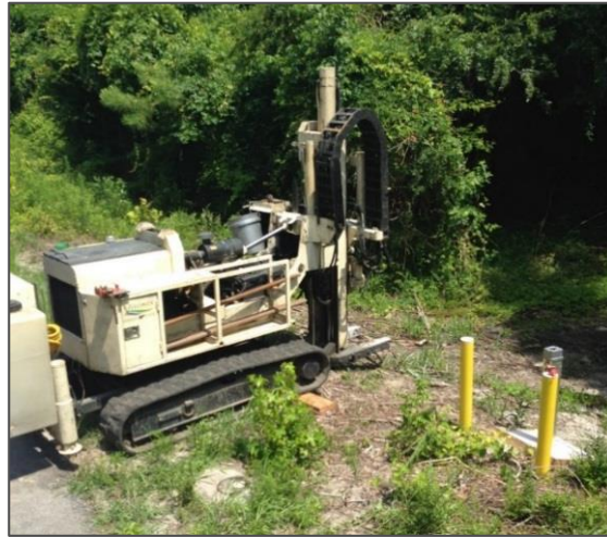
Substrate, bioaugmentation culture, and red yeast rice (RYR) injections
