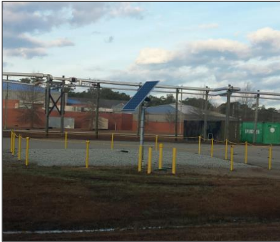
Solar-powered subgrade biogeochemical reactor (SBGR)
