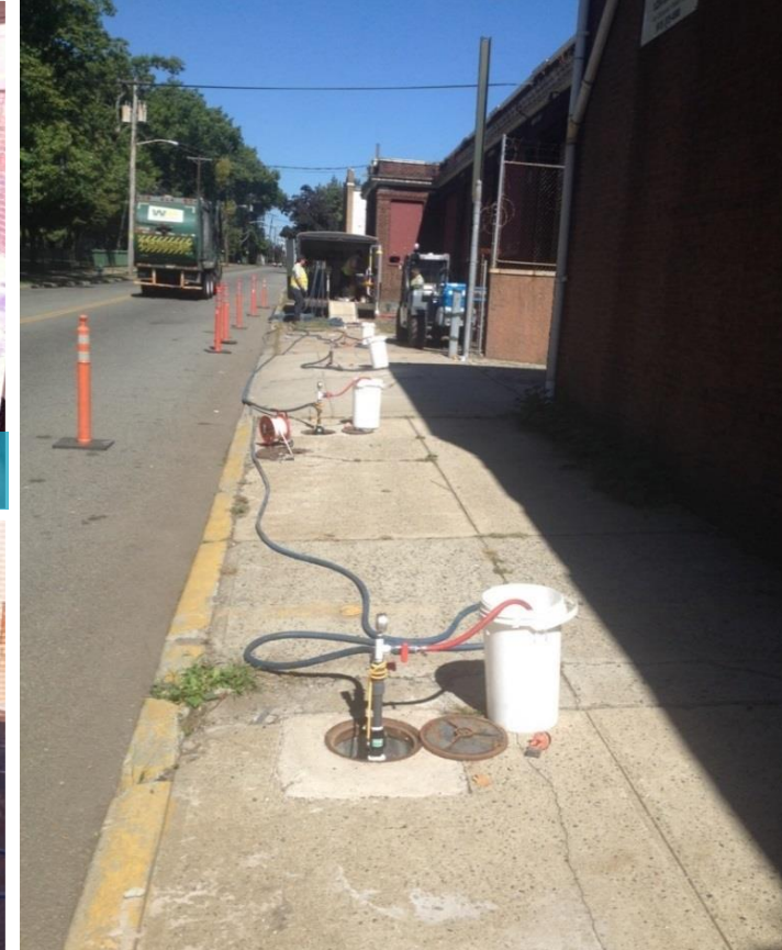
Biobarrier injections
