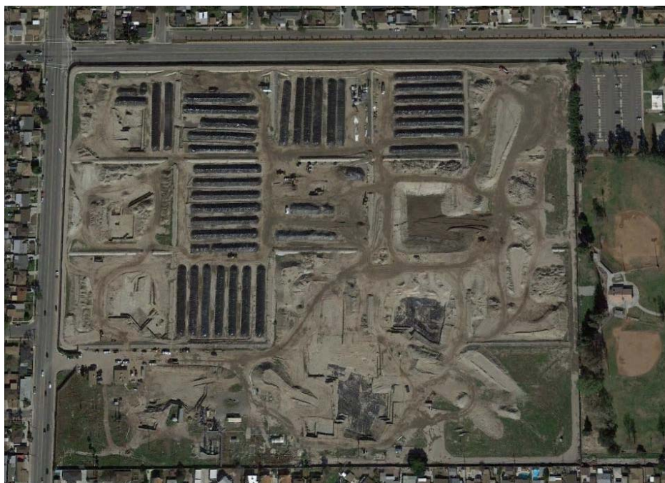
FIGURE 1. Former Department of Defense bulk fuel distribution facility.
