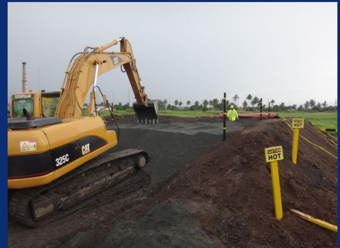
Placing Clean Cover Material
