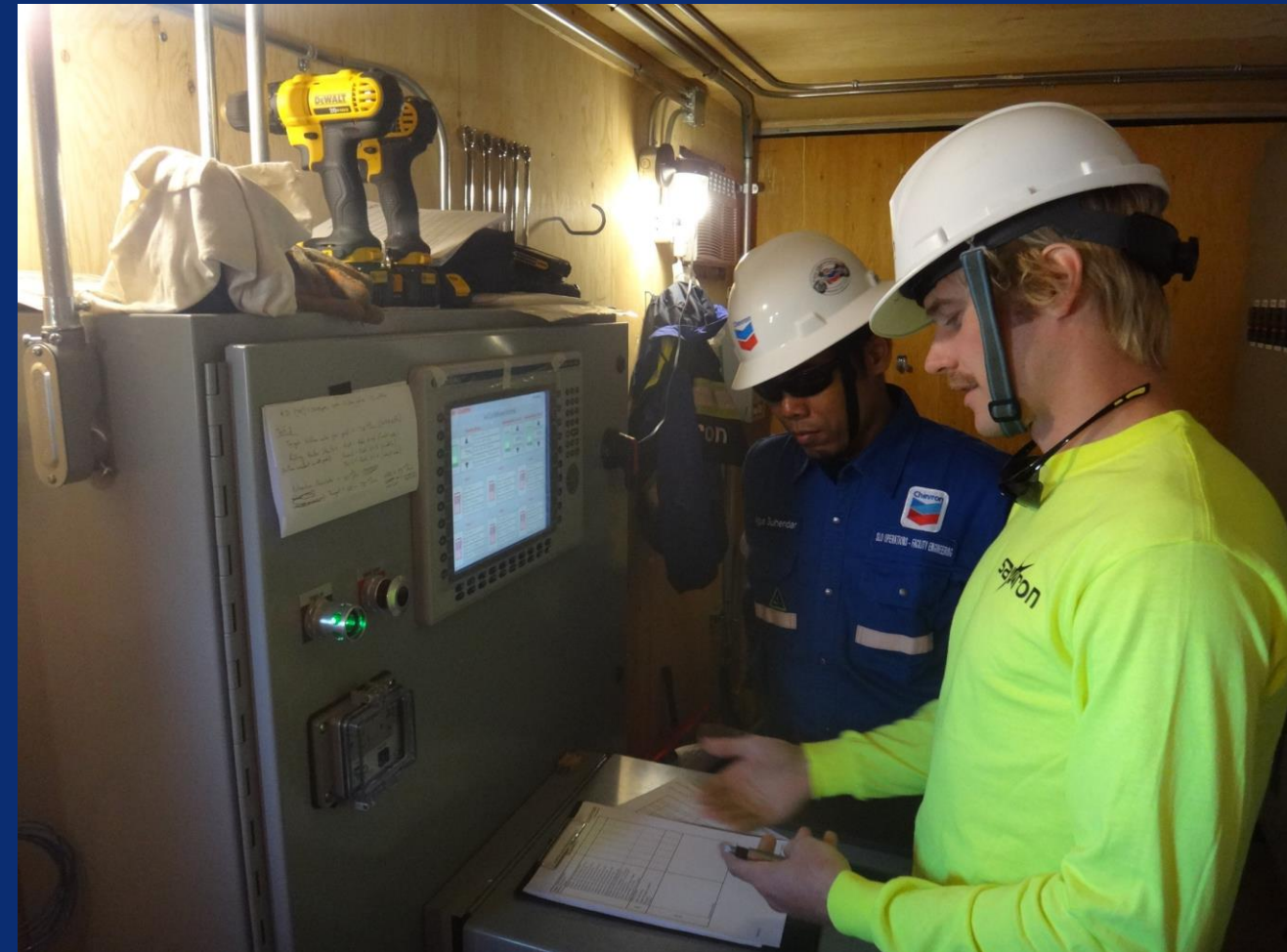
Main Control Panel
