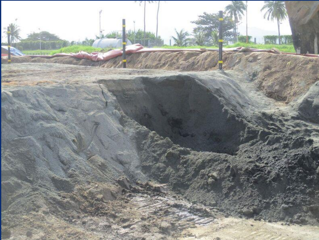
Removing Clean Cover Material
