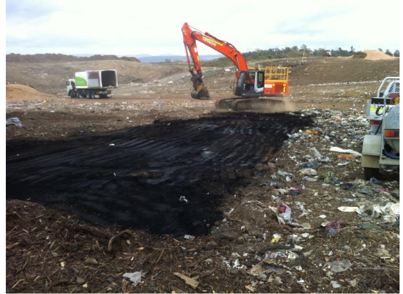
Finished lined burial cell
