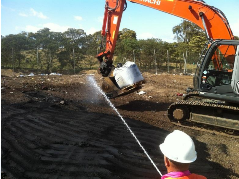
Laying the RemBind capping layer
