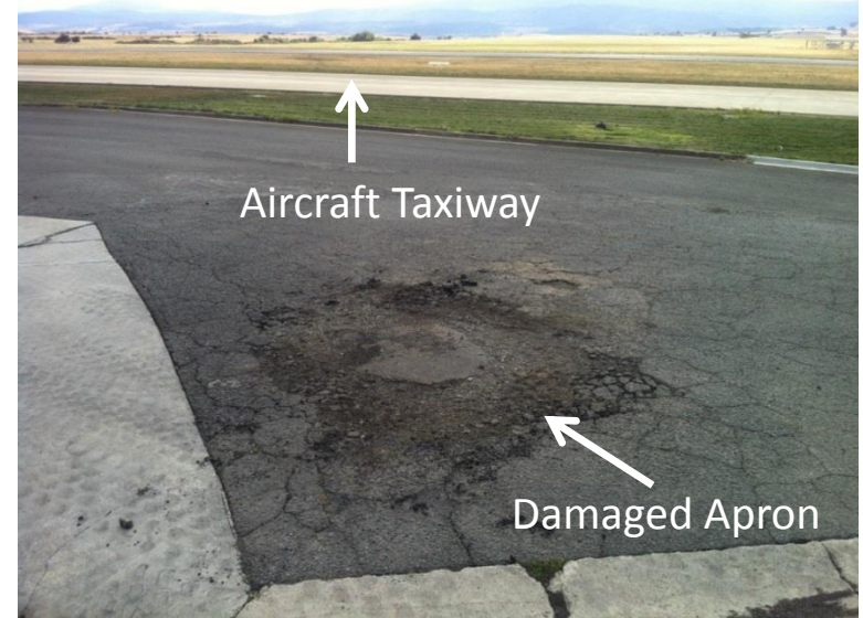
Damaged asphalt apron
