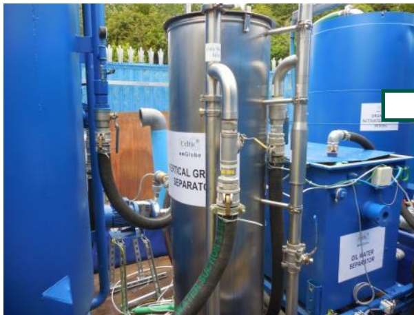
Oil / Water Separator & Silt Trap
