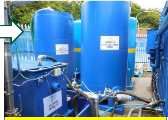
Vapour Phase GACS and Vent Stack
