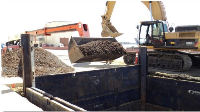
Source Area Excavation/Backfill
