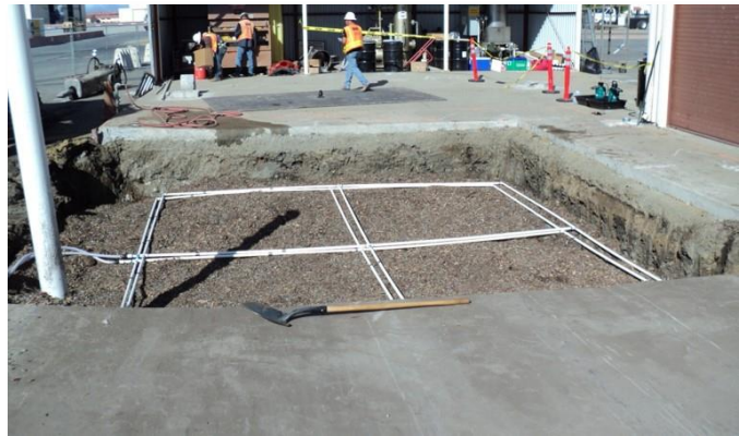
Infiltration Pipe Installation
