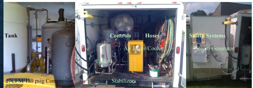
Feed Systems, Safety Systems, Compressed Gas Systems All piping Welded Stainless Steel Floors Coated in Chemical Resistant RinoLining
