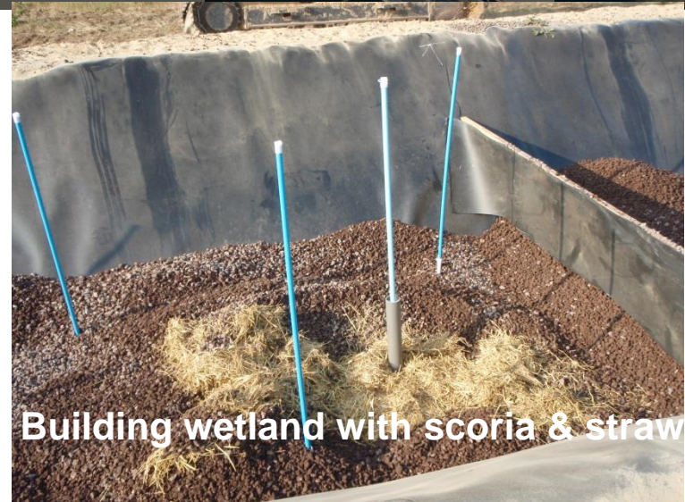
Placing liner and maintenance drain
