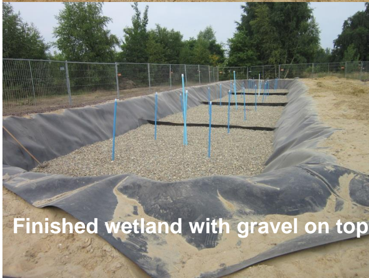
Placing liner and maintenance drain
