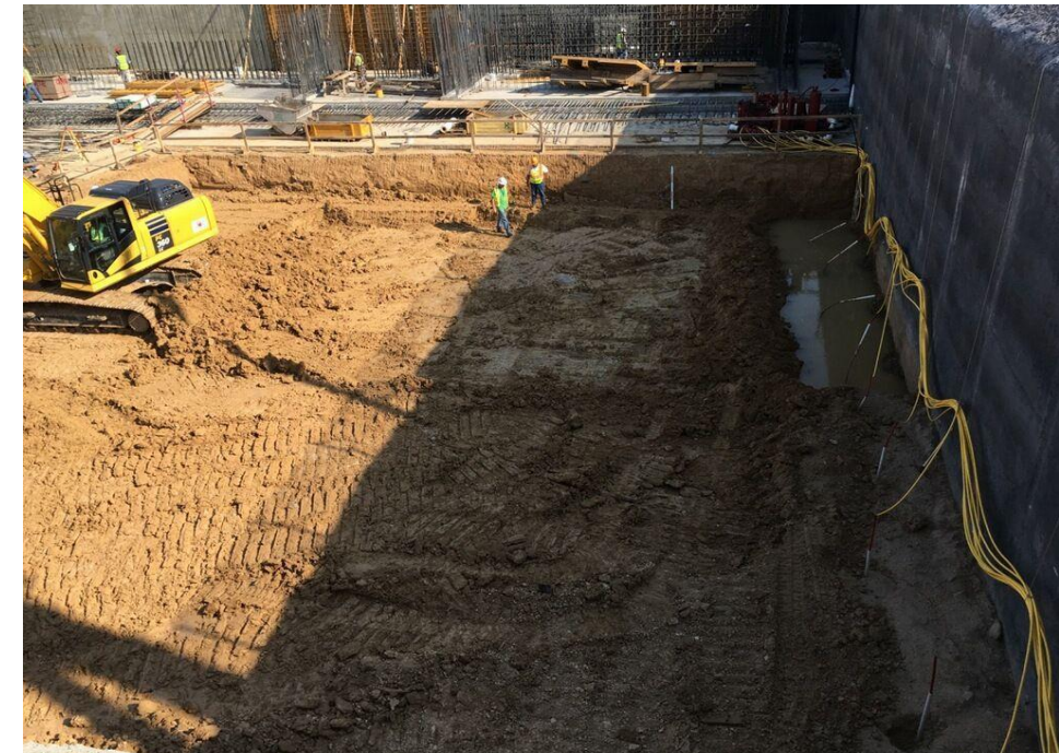
Over-Excavation of Pond Bottom
