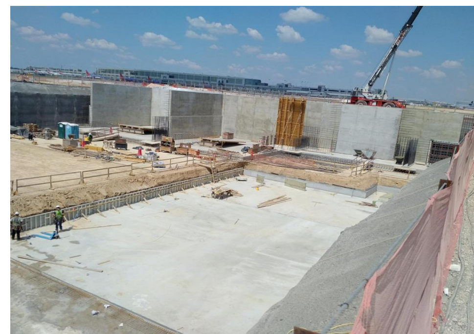
Concrete Installed Over Flowable Fill
