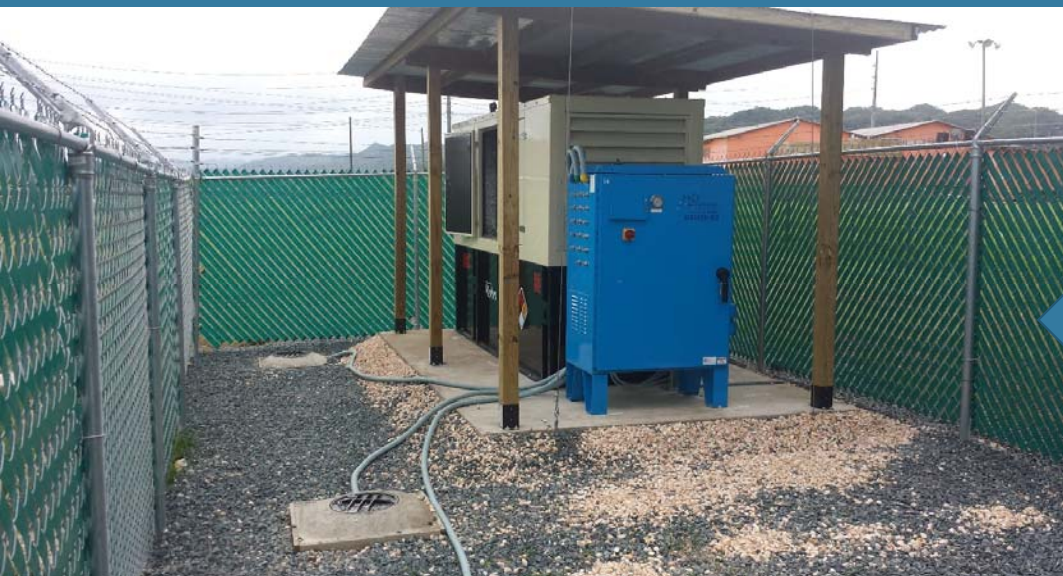
Inside Compound Ozone Sparge Wells
