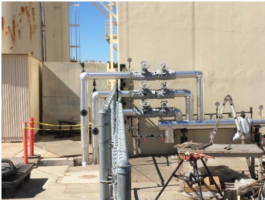
Steam Injection Manifold
