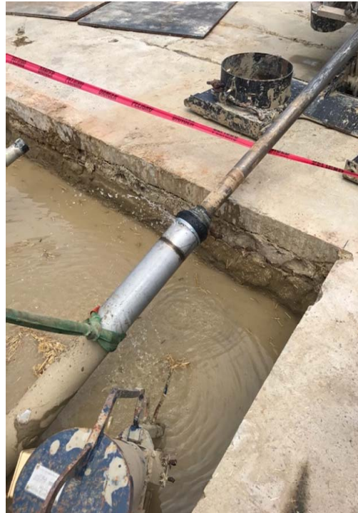
Horizontal Well – The Beginning.....
