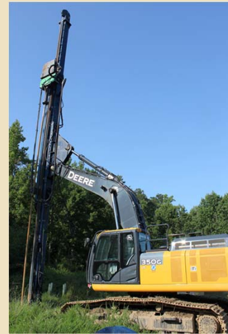
Pump amendment up mast and into mandrel for emplacement
