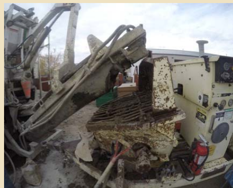
Deliver amendment into hopper and displacement pump
