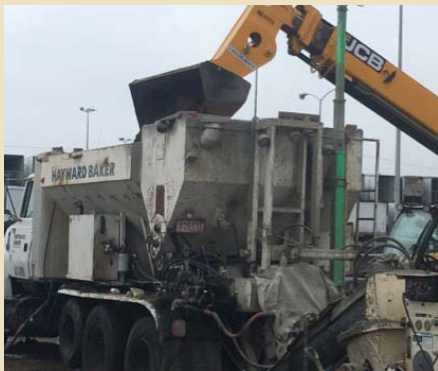
Batch-mix amendment ingredients in Elkin Mixer
