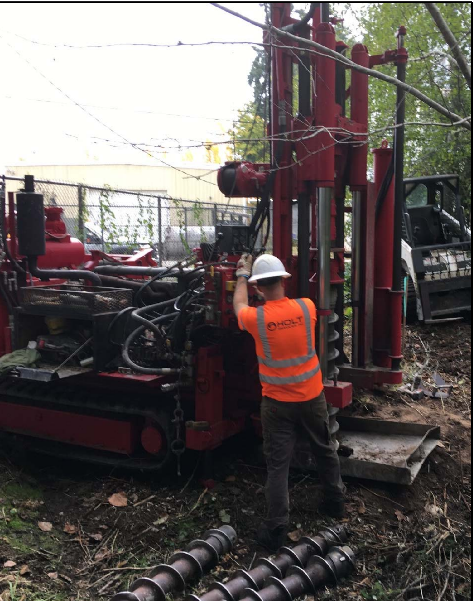
Installing new permanent monitoring wells based on the results of high resolution site characterization.
