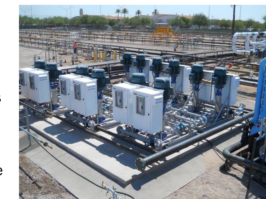
Installed SEE treatment system
