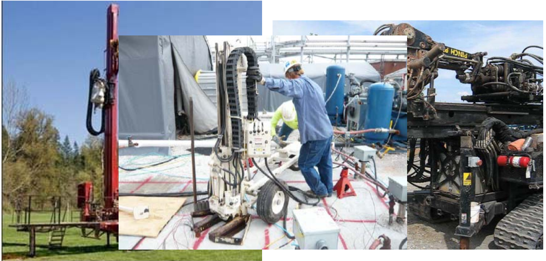
ERH electrode installation (10-14")
