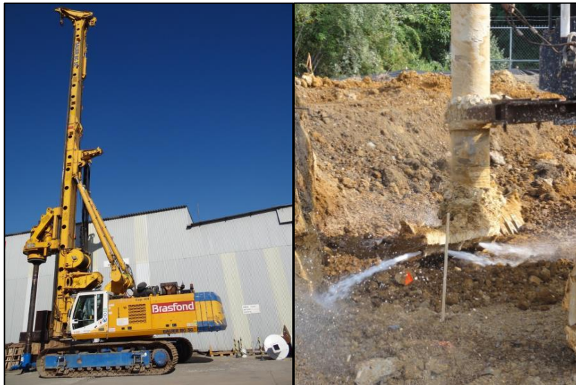
FIGURE 2. Drill rig & large diameter auger
