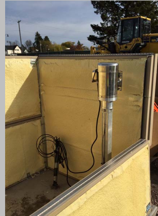
Anchor Electric pumping in Ashland residential neighborhood
