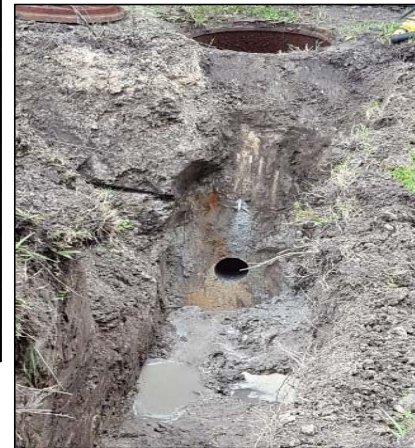
Blower Connection to Manhole
