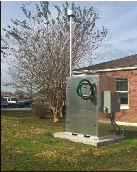
Blower Enclosure and Stack
