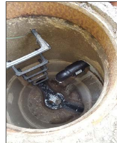
Blower Connection to Manhole
