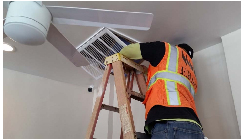
Placing new filter in new intake
