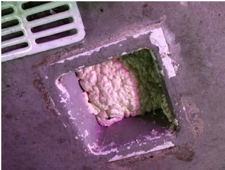
Sealing floor drain
