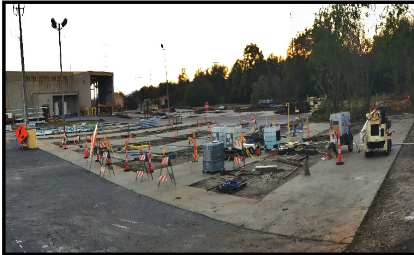
20 to 30 simultaneous DPT injection locations through an active facility
