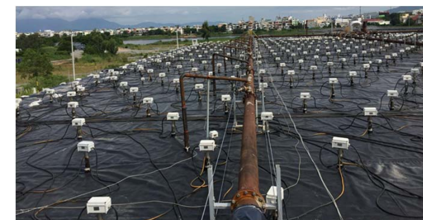
Completed surface – Phase 2
