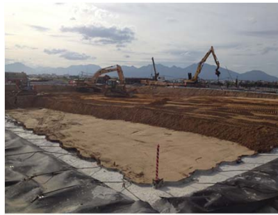
IPTD ® pile construction & filling
