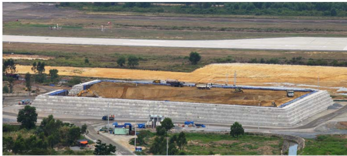
IPTD ® pile construction & filling
