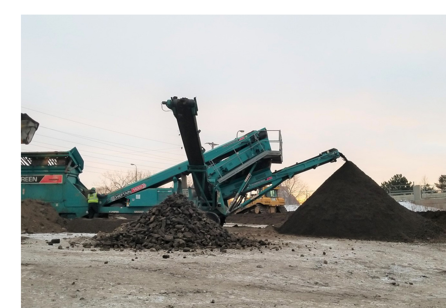
soil screening equipment removed debris from soils that were reused on-site
