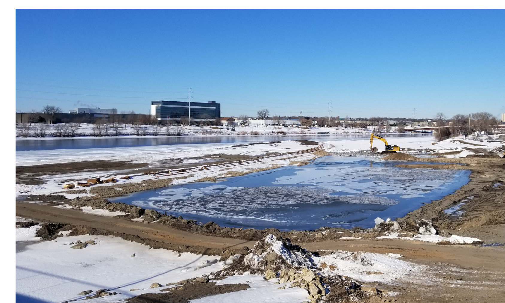
land bridges were used to contain suspended sediments and for truck and excavator traffic during construction
