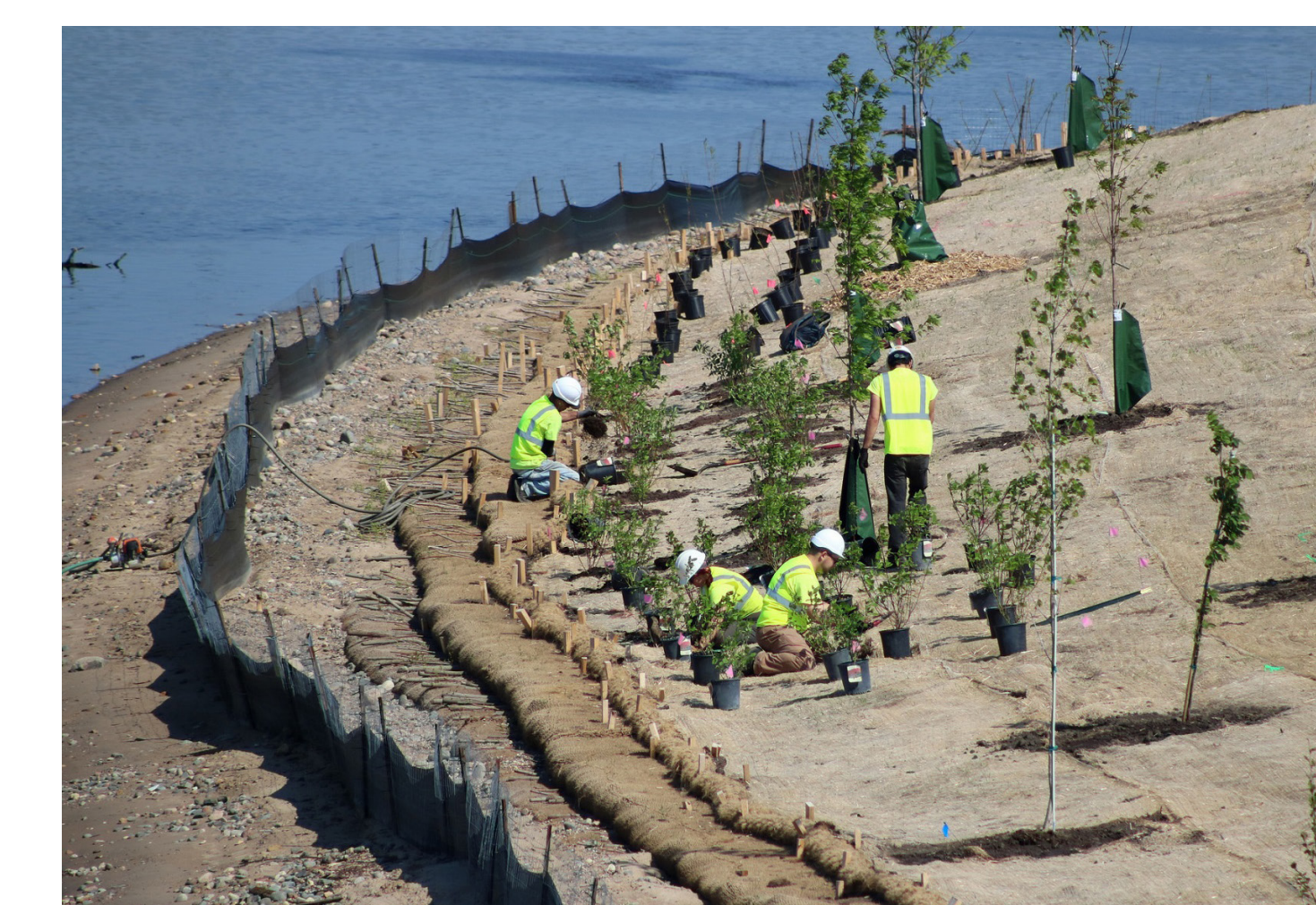
planting of trees, shrubs and willow stakes on the riparian bench (photo credit: MWMO)
