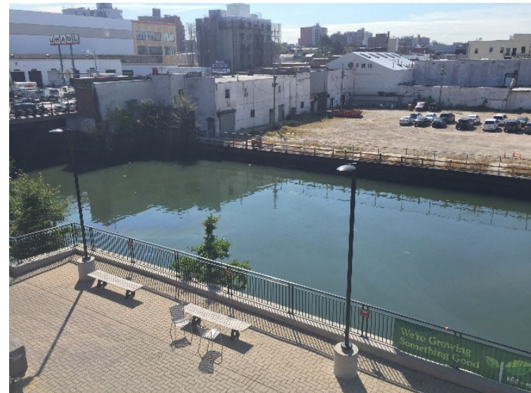
4 th St. Turning Basin (looking South)
