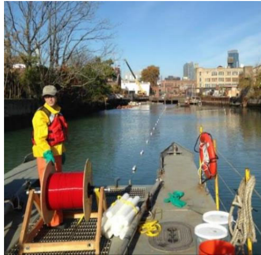
Fiber Optic Cable Installation - Temperatures
