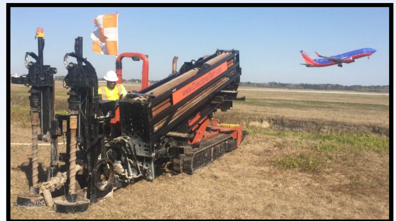
Installing first ever horizontal remediation wells (HRWs) in South Korea
