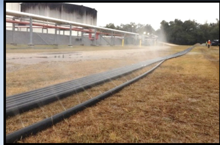
Water being pumped through horizontal remediation well to demonstrate uniform flow through well screen
