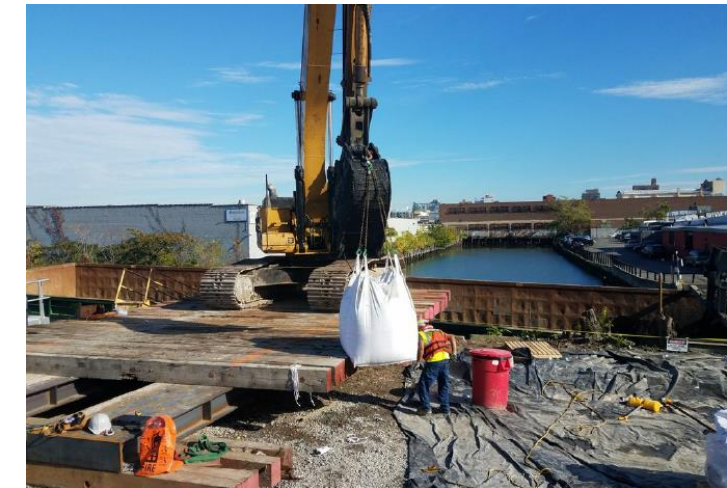
FIGURE 2: Supersack of Portland cement ready for mixing into dredged material.
