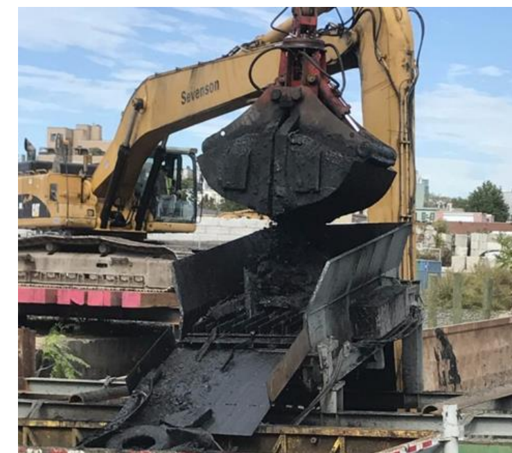
FIGURE 5: Dredge material passing through onsite vibratory grizzly screen to separate oversized debris from sediment.
