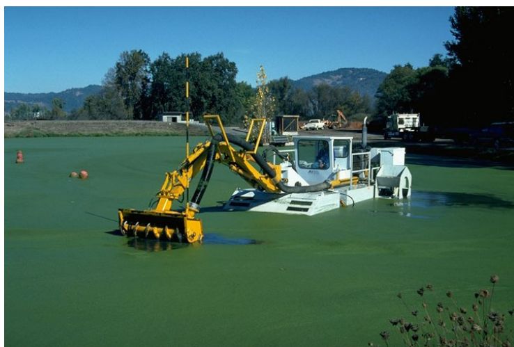
Approach I - Tilling in Bioamended SediMite to access PCBs at bottom
