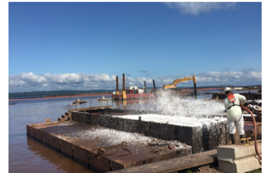
Apply Rusmar Foam - control odor
