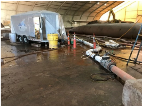
Chemical dosing dredge feed
