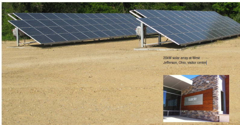
Battelle's Net Zero Energy Visitors Center is equipped with a solar array and geothermal system
