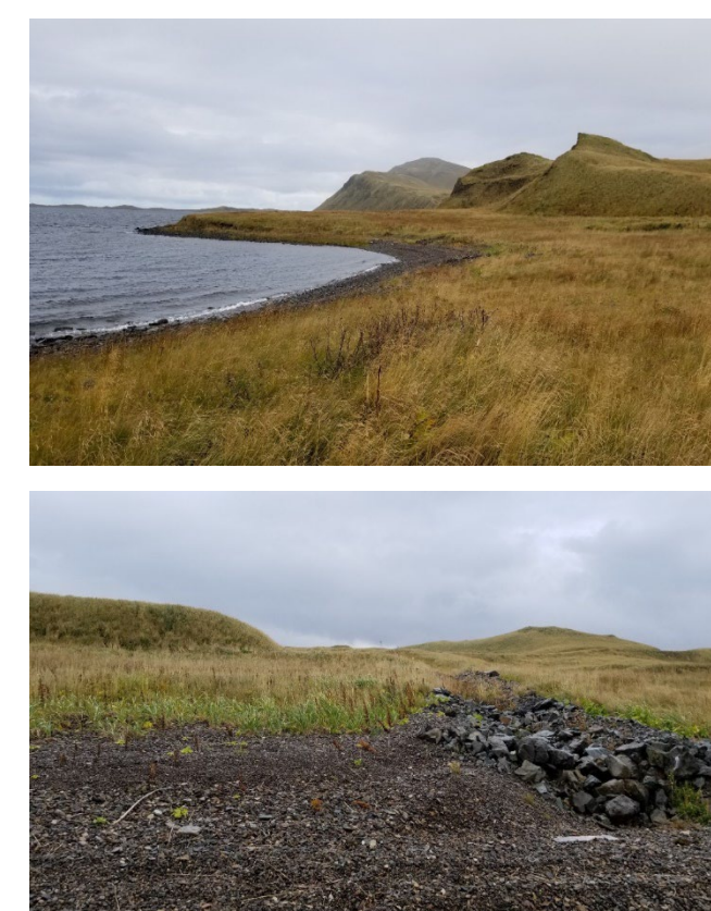
Figure 3. Views of the SWMU 4 Landfill
