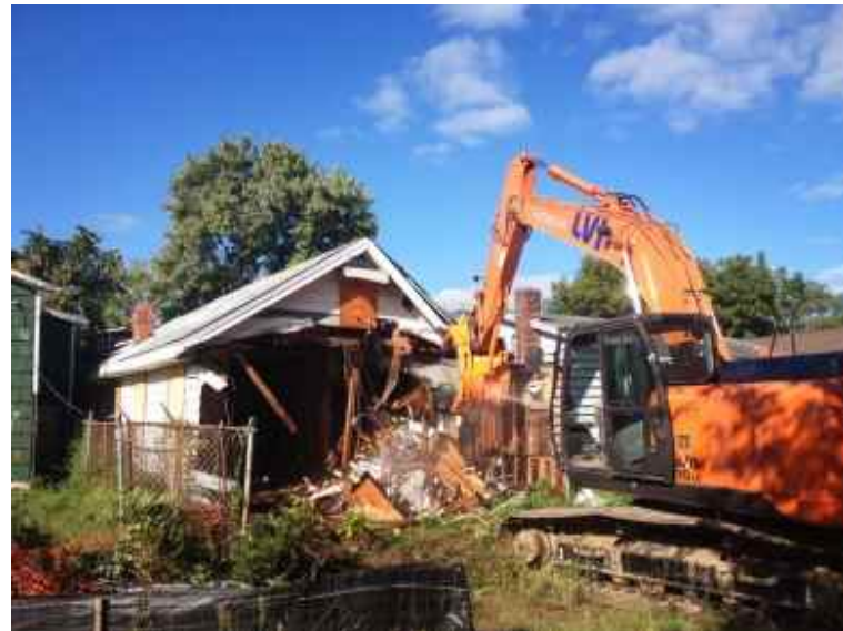
Demolishing a home flooded by Sandy
