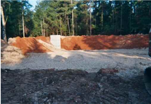
Constructed pond/wetland closed-loop recirculation system during installation
