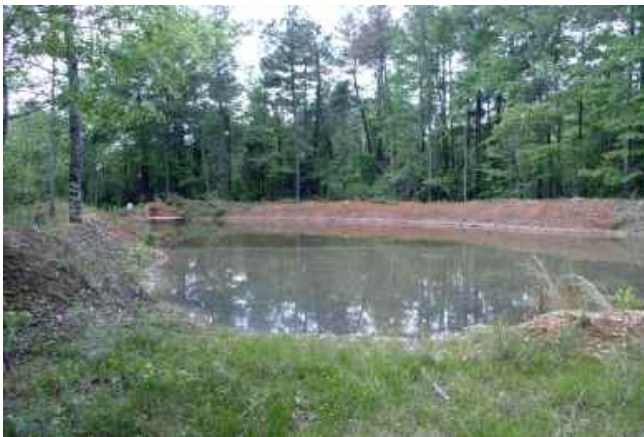
Constructed pond/wetland closed-loop recirculation system 1 year after installation
