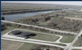
1999 Liquid Tank Terminals
